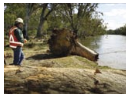
Re-snagging involves large machinery to place large hardwood logs.
