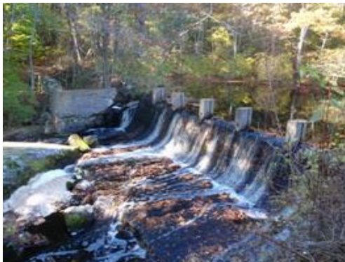
The Tack Factory Dam as it was. Photo: NOAA
