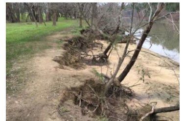
This type of bank erosion on the River Murray is typical of that caused by boat wash. Photo: Ben Berry.
