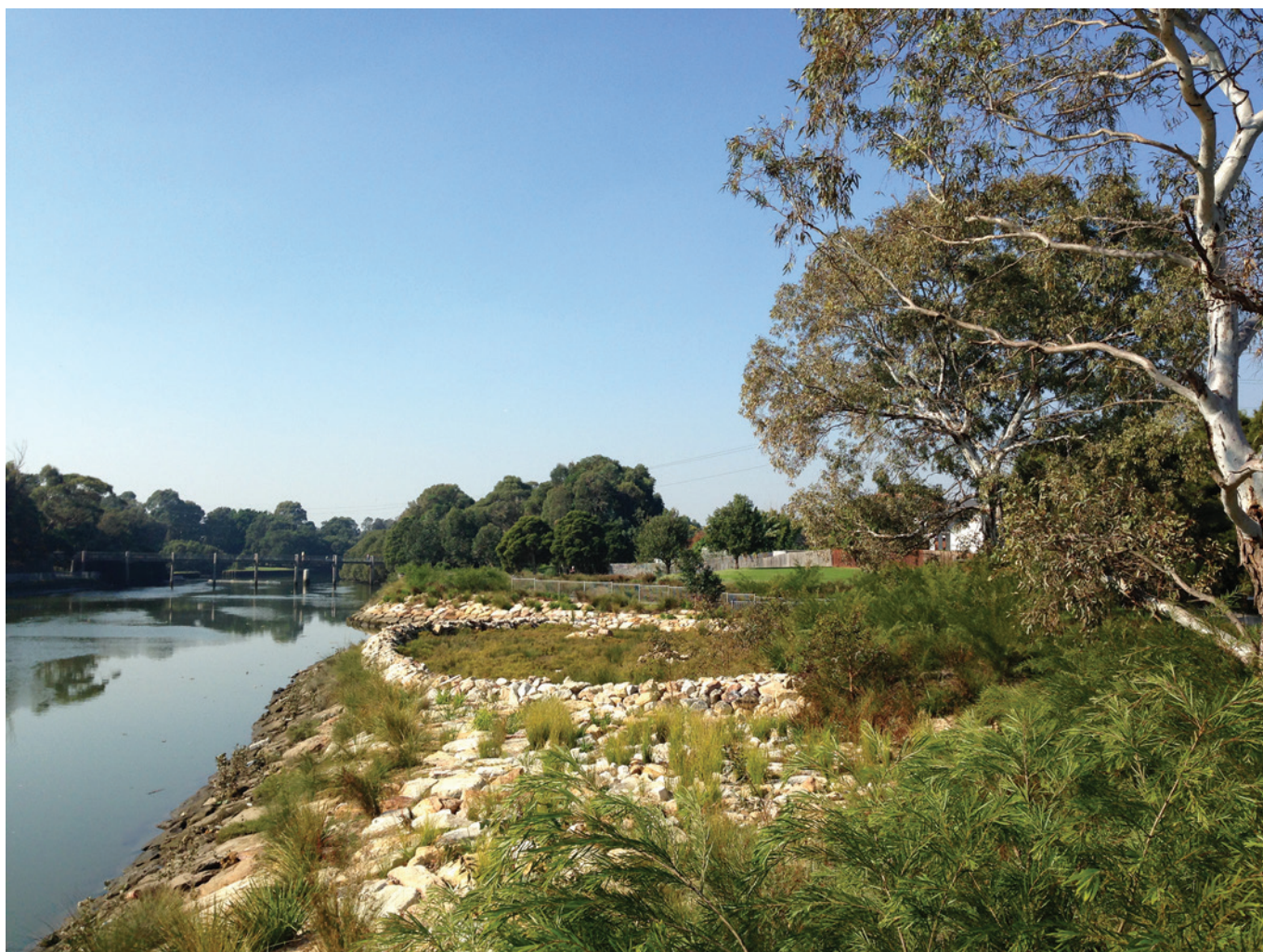
Figure 6. Riparian reed plantings in foreground, saltmarsh bench in background, looking downstream.
