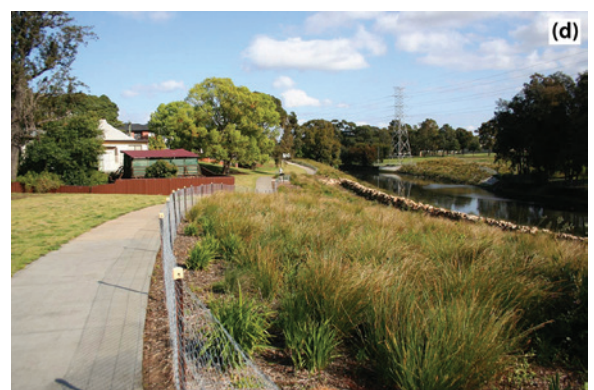
Figure 4. Drain naturalisation process from concept design (a) to action on the ground (b, c) and the newly remediated site (d).
