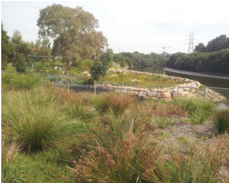
Figure 1. Riparian revegetation (foreground) and saltmarsh bench (background) at Cup and Saucer Creek.
