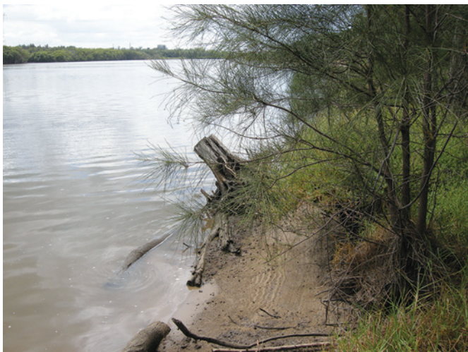
Figure 8. a) Photo point 7, undercut banks, failing riparian vegetation before works, 2011.
