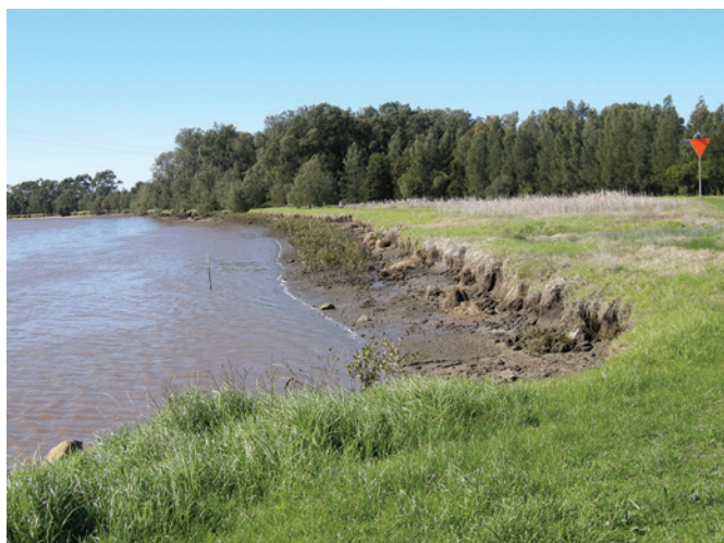
Figure 9. a) Photo point 4 before works March 2010, vertical banks and at risk mangrove recruitment.
