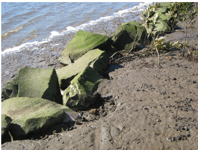
c) Sediment deposition and minor rill erosion at low fillets following minor flood.
