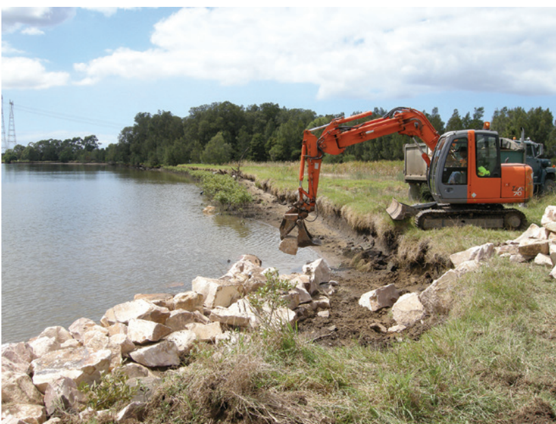
Figure 6. Rock fillet construction underway.
