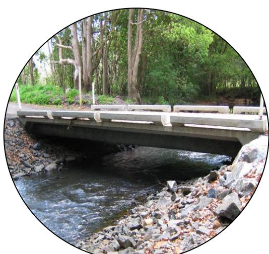
**IMPROVE ROAD CROSSINGS\*** - Where box culverts replaced three pipe culverts, monitoring showed reduced water velocities and improved fish passage by 14 - 44%.
