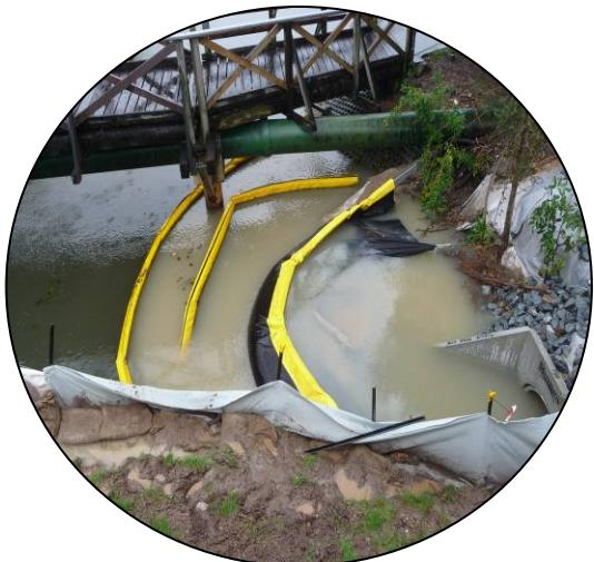
Encourage your council to be a **FISH FRIENDLY COUNCIL** - control erosion and siltation at work sites like this silt curtain being used at Banora Point (Tweed Heads).
