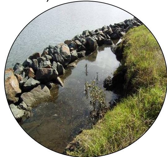
Help install **ROCK FILLETS\*** like these protecting the Wallamba River bank from wave induced erosion on the.
