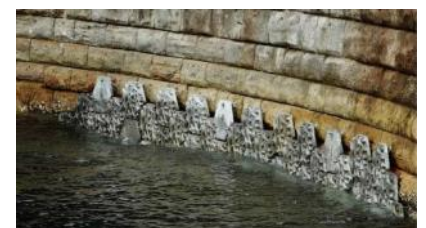
An area of seawall with the tiles installed. Photo: Hollie Adams.
