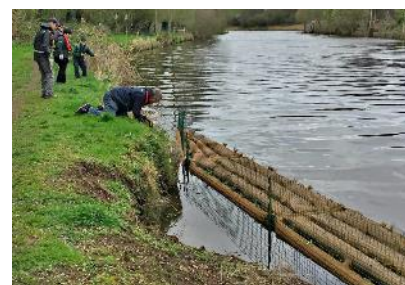
Floating habitats installed on the River Weaver to river wildlife and improve water quality. Photo: The Environment Agency UK.
