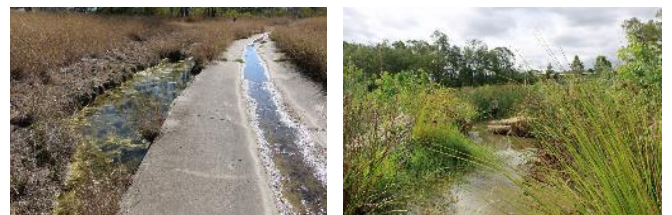
Small Creek had been converted into a concrete channel (left) but is now being restored (right), and the fish are making their way upstream from the Bremer River. Photos: Ipswich City Council.
