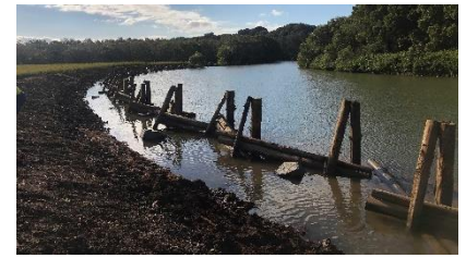
A complex log fillet design to address erosion and support the return of mangroves. Photo: North Coast Local Land Services.
