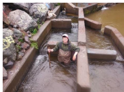
The cleaned up fishway. Photo: SaltWire Network.
