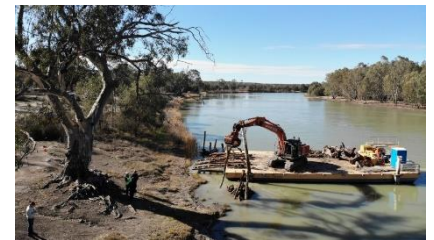
Increasing the density of snags to 'fish up' earlier resnagging efforts in a denuded stretch of the River Murray. Photo: SA Department of Environment.
