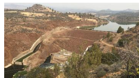
At 173ft (53m) high, the Iron Gate Dam is the largest dam set to come down on the Klamath River. Photo: Dave Meurer.
