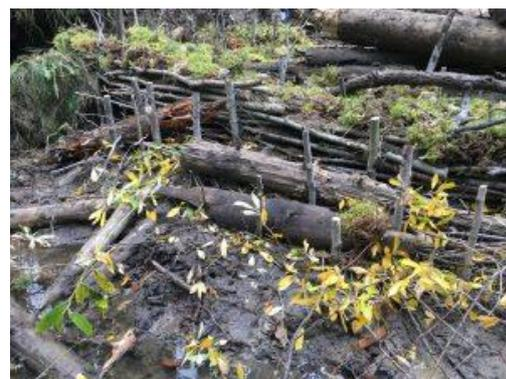
A variety of bioengineering techniques, such as willow staking, willow wattle fences, log walls, and seeding was used to improve bank stability and reclaim stream crossings. Photo: Trout Unlimited Canada.
