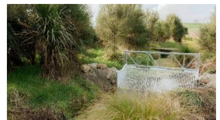
The design of this barrier enables native fish and eels to enter the lake but not Koi. Photo: Waikato Times.
