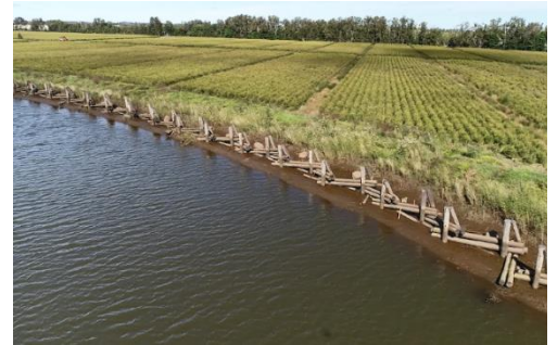
Log fillets protect a newly formed mangrove nursery from boat wave wash. Photo: North Coast Local Land Services.
