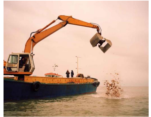
Tonnes of shellfish shells are dropped at a time, gradually rebuilding what was once a flourishing oyster reef. Photo: Jacob Dykes.
