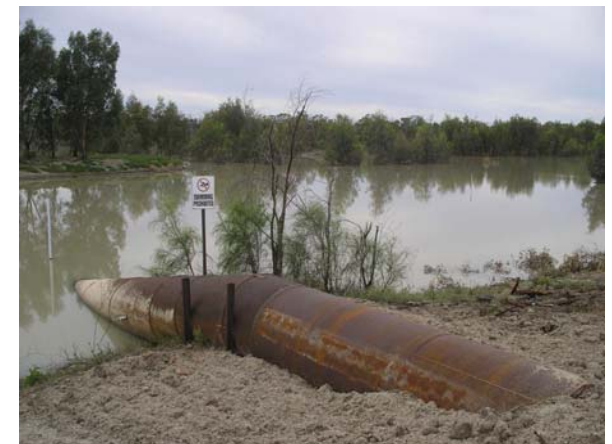
Irrigation offtake Tandou Creek. Photo: Scott Nichols.
