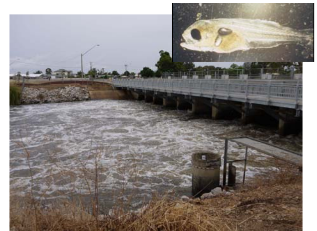
Downstream of the Mulwala Irrigation Canal inlet regulator. Native fish larvae (pictured) are mostly killed when they go through this type of structure. Photo: Jodi Frawley. Larva photo: Lee Baumgartner.
