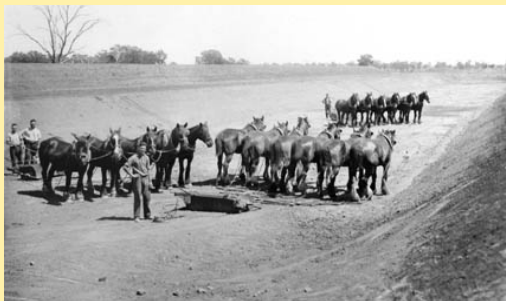
Building the canals was hard work but provided welcome employment during the Depression. Photo source: http://www.irrigationhistory.net.au/ .
