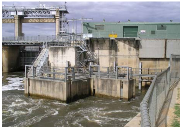
Encased in all this concrete is a 'vertical slot fishway' that allows larger migratory fish like Murray cod, trout cod, golden perch and silver perch to migrate past Yarrowonga Weir. Photo: Scott Nichols.
