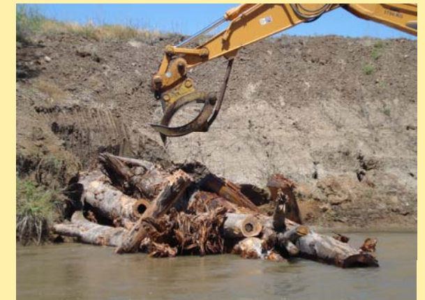
The construction of a log groyne involves a lot of analysis, planning and getting appropriate permits – all before a log enters the water. It's so much easier if it happens naturally! Photo: Milly Hobson.
