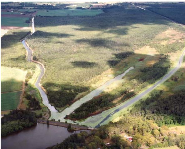
Tuckean Swamp on the Richmond River was a tidal wetland. When the barrage, lower left, was constructed in the early 1970s it restricted saltwater flows. By 1989 306 hectares of mangroves and 134 hectares of saltmarsh had been lost. Image I&I NSW.
