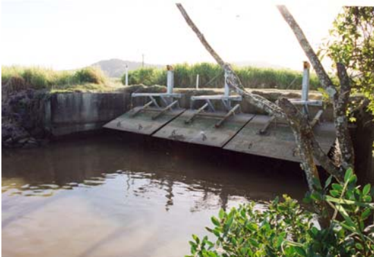
Actively managed winch gates can be fully removed from the water.
