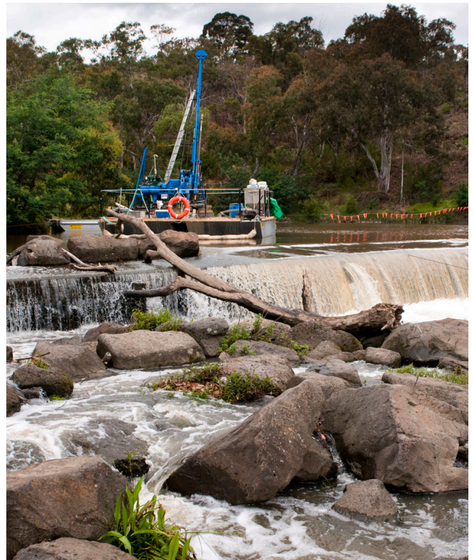
Geotechnical investigations at Dights Falls, 2009
