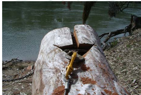
Photo 2: A cut is made in the log for the metal plate, to which the cable is attached. Photo: Jenny Fredrickson
