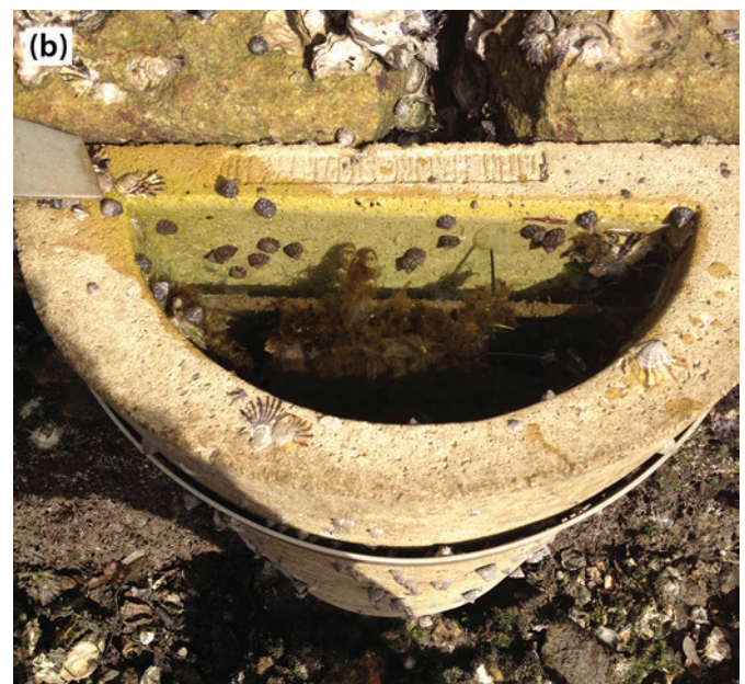
Figure 2. Complex tiles (a, left) and flowerpots (b, right), retrofitted to seawalls to mimic important microhabitats of rocky shores which are missing or rare in existing seawall designs of Sydney Harbour.
