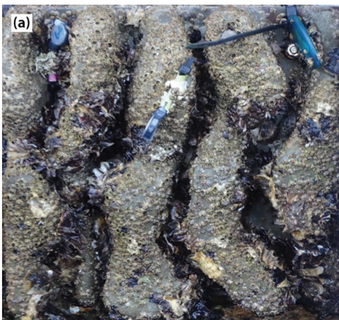
Figure 2. Complex tiles (a, left) and flowerpots (b, right), retrofitted to seawalls to mimic important microhabitats of rocky shores which are missing or rare in existing seawall designs of Sydney Harbour.
