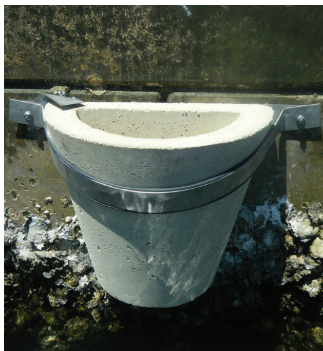
Figure 4. Flowerpots were constructed by Antique Stone and attached to the seawall using stainless steel brackets.
