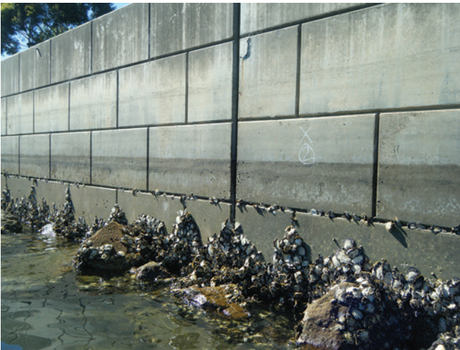
Figure 1. a) Example of a typical seawall.
