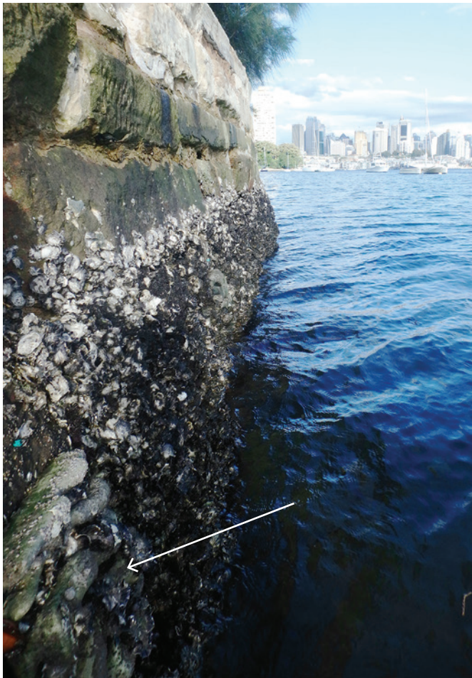
Figure 5. Complex tiles in-situ (bottom left corner) retrofitted to a seawall.
