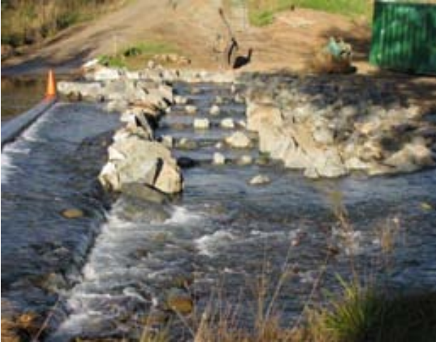
Partial width rockramp at Kings Crossing on the Bowman River. Photo: Shaun Morris
