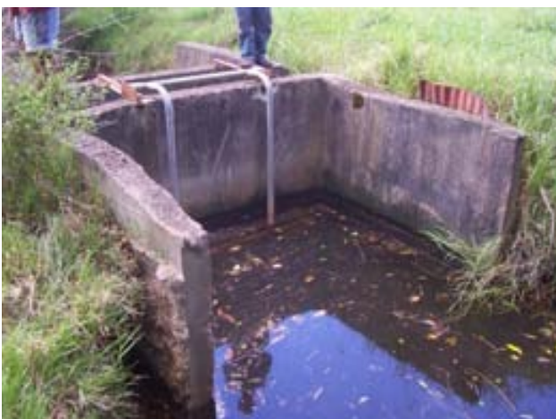
Out with the old floodgate.....
