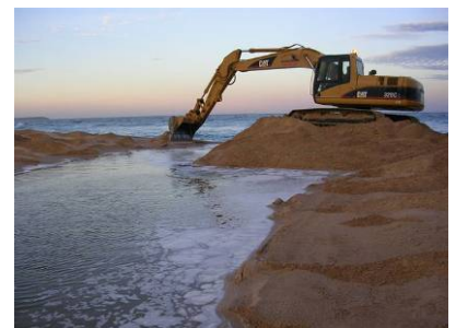
The use of heavy machinery to artificially open ICOLLs is subject to guidelines. Image: R Massie
