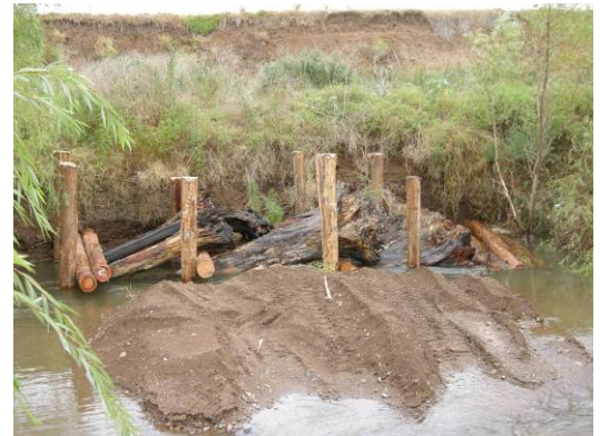
One of the log jams prior to being covered with gravel. Photo: Kylie Russell
