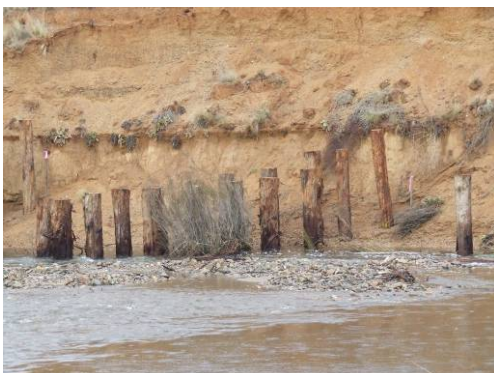
One of the 'pin sets' installed to help control bank erosion on the Numeralla River. Photo: Charlie Carruthers.
