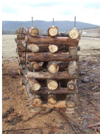
Hardwood timber cribs were placed between the pin-sets to protect the eroding bank and increase the deposition of suspended sediment from the water column. Photo: Charlie Carruthers.
