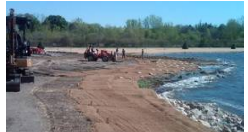
As part of the project, 10,000 feet of hardened shoreline is being replaced with native vegetation. Photo: Structurespot.com.
