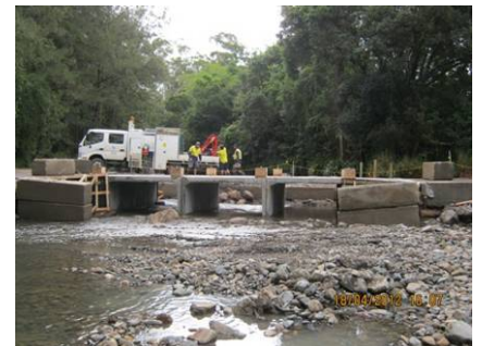
One culvert might look the same as another to us, but 'thinking like a fish' puts these functional structures in a new light. The new culverts on the Dungay Creek crossing (above, photo: Kempsey Shire Council) and on the Yass River (below, photo: Yass Valley Council.)
