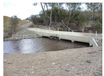
One culvert might look the same as another to us, but 'thinking like a fish' puts these functional structures in a new light. The new culverts on the Dungay Creek crossing (above, photo: Kempsey Shire Council) and on the Yass River (below, photo: Yass Valley Council.)
