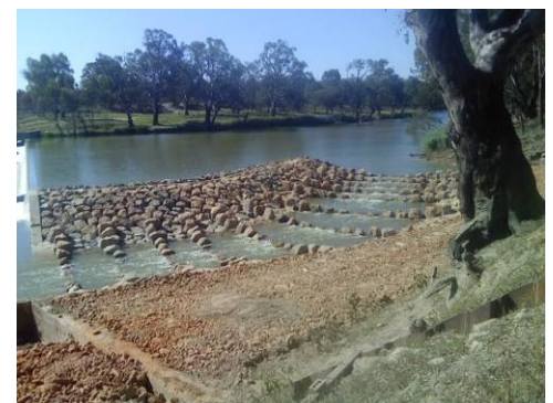
The completed fishway on the Brewarrina weir. Photo: David Cordina
