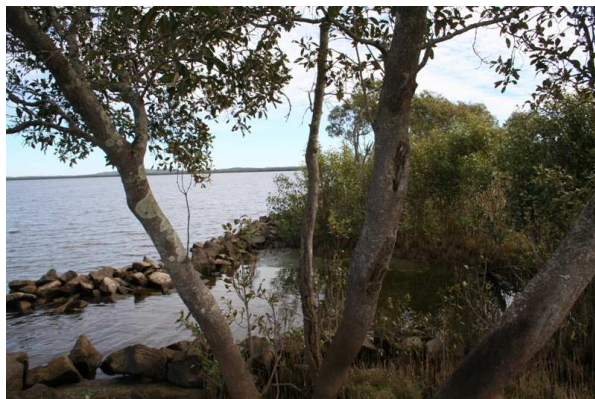
Some of rock fillets on the Lake Wooloweyah foreshore (left) and an example of successful accumulation of sediment and juvenile mangroves behind a rock fillet established in 2006 (right). Photos: Pat Dwyer.
