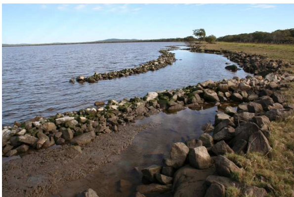
Some of rock fillets on the Lake Wooloweyah foreshore (left) and an example of successful accumulation of sediment and juvenile mangroves behind a rock fillet established in 2006 (right). Photos: Pat Dwyer.
