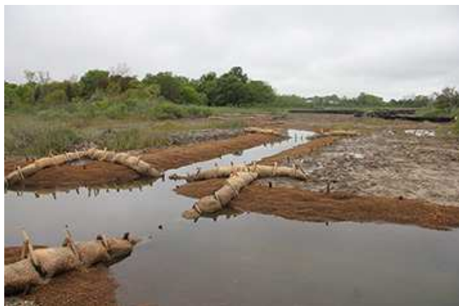
The reconstruction of tidal creeks is improving the flow of tidal water and enabling the establishment of saltmarsh vegetation. Photo: NOAA/Restoration Center/Howard Schnabolk
