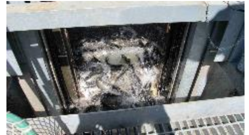
Alewives in one of the fish lifts. This past Spring 2.1 million Alewives were lifted over the Benton Falls dam. Photo: Rick Lawrence
