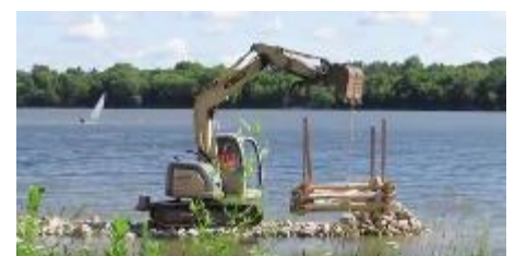
Fish 'cribs' were the first stage of the creation of more fish habitat. Photo: Upper Thames River Conservation Authority.
