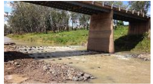
The Condamine Town Weir fishway. Image: Queensland Country Life.
