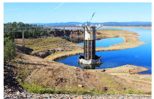
A thermal curtain directs warmer surface water to the tower outlet. Photo: Guresh Ahuja.
