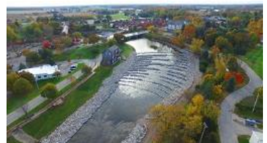
The new 350m rock ramp fishway lets fish access habitat upstream of Frankenmuth Dam for the first time in 150 years. Photo: U.S. Army Corps of Engineers
