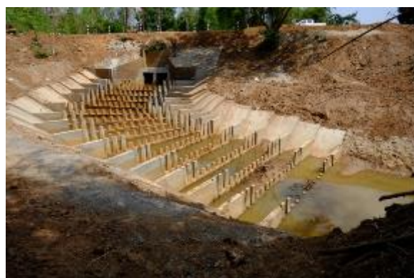
Before (left) and after (right) the construction of the fishway on a tributary of the Mekong River, Laos. Photo: ACIAR
