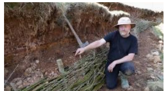
Willow spiling is an old technique used to control riverbank erosion. Image from video: West Cumbria Rivers Trust
