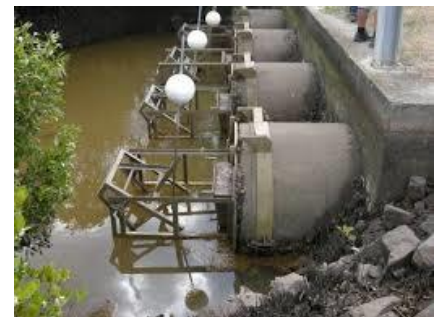
An example of a tidal floodgate operating in the Hunter estuary. Photo: NSW DPI.
