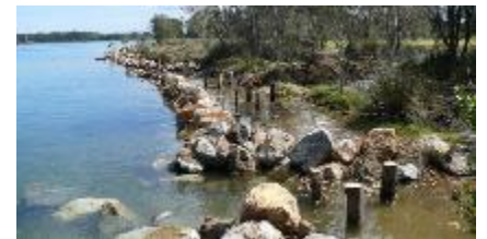
Estuarine restoration using timber and rocks from nearby road works. Photo: NSW OEH.
