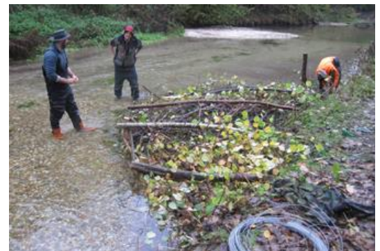
Creating woody mattresses, using material from the opening up of the canopy, was part of the rehabilitation of fish habitat on the River Dever. Photo: Wild Trout Trust.
