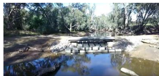
A perforated metal grate on the surface and baffles to slow water underneath mean that these new bridges enable fish to migrate in a variety of conditions. Photo: NECMA.
