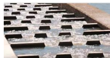
The new cone style fishway at the Rockhampton Barrage is now seeing over 400 fish a minute bypass the barrier. Photo: Extracted from video, Fitzroy Basin association.
