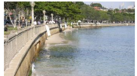
Woollahra Seawall – not a fish friendly structure. Photo: NSW DPI.
