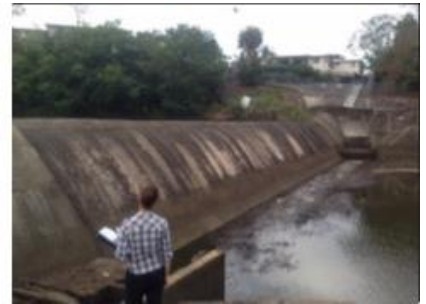
Caboolture Weir is the top-ranked barrier to fish passage in SE QLD. It is estimated that a bypass rock-ramp fishway could remediate this barrier for under $250k. Source: Catchment Solutions.
