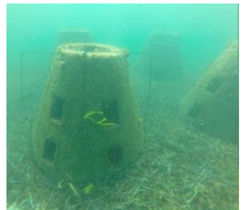
One of the structures that make up the artificial reef at Port Coogee. Photo: Subcon.
