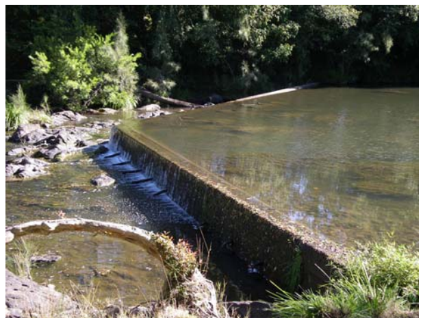
Stroud Weir, a 1 m high structure on the Karuah River, restricted fish migration to over 70 km of upstream habitat.
