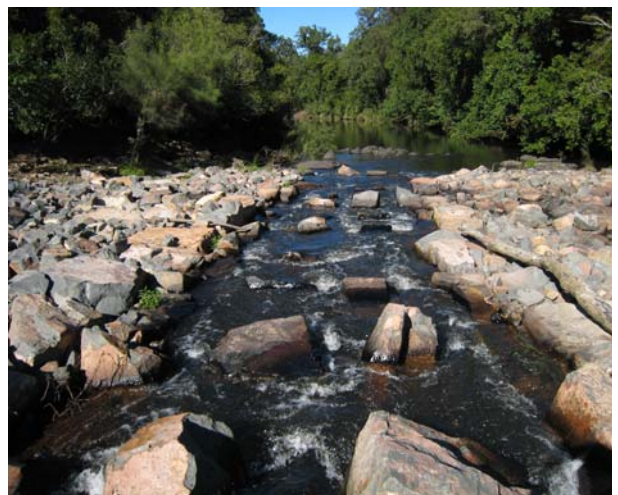
Access for fish was reinstated at Stroud Weir with the construction of a rock ramp fishway.
